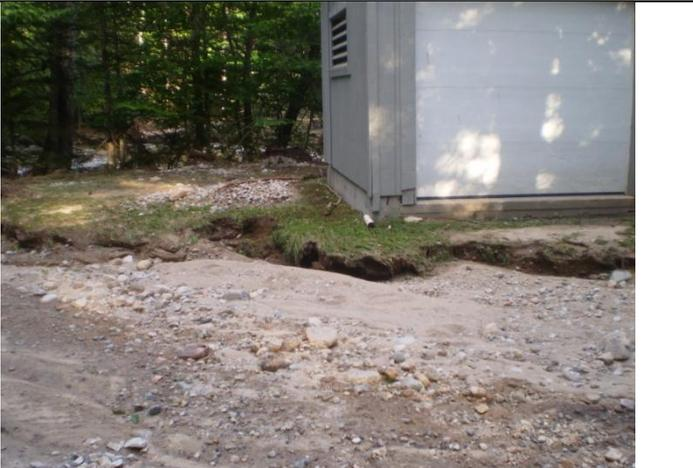
A photograph showing a grey metal pump house with significant erosion at its base. The ground in front of the building is a mix of dirt and rocks, with a deep channel of water or mud running alongside it.              | <p>Pump House #1 Erosion<br/>Taken on 08/29/11</p>  |
